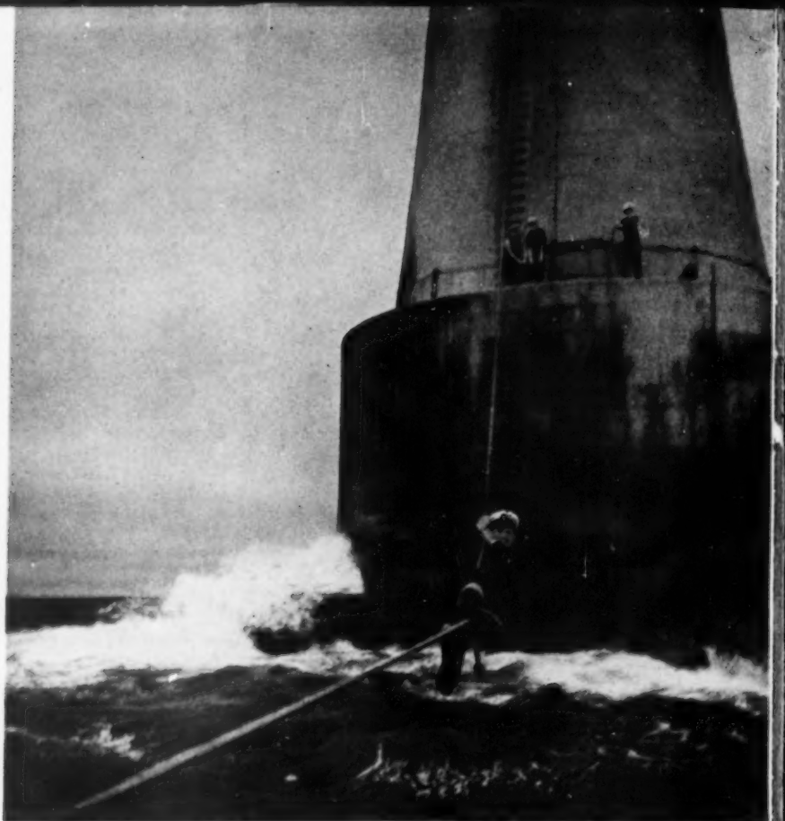
Commuting to work. A keeper clings to the bowline which is carrying him up from the relief boat to the landing platform of the lighthouse.
